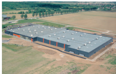
THK Manufacturing of Europe S.A.S.(FRANCE) Site: 198,559 m 2 (2,137,289 sq.ft.) Floor space: 32,484 m 2 (349,658sq.ft.) Fläche: 198.559 m 2 , Gebäude: 32.484 m 2
